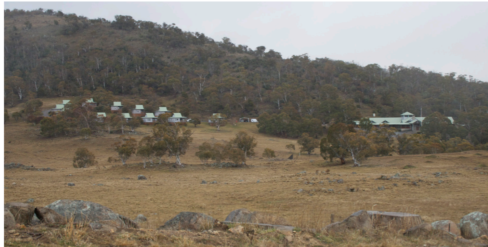
Figure 19 Jindabyne locality accommodation buildings in landscape setting
