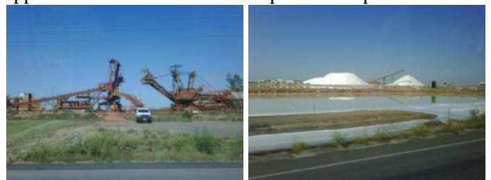
Industrial landscape, Pilbara Region, WA
